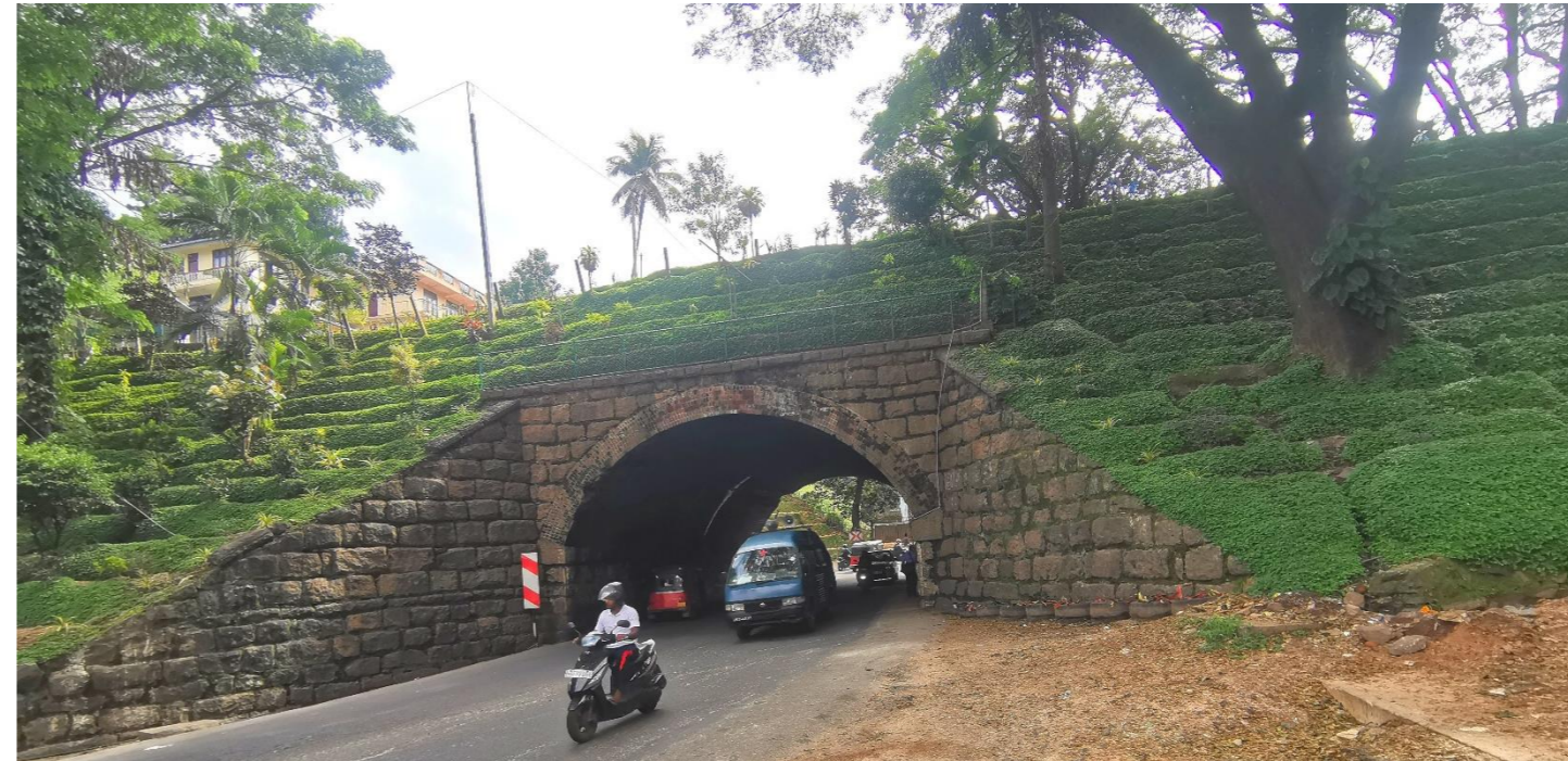
Figure 30: Mahayyawa Tunnel - Existing Situation
