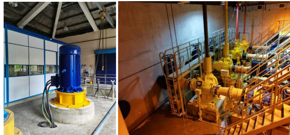
Figure 44: Intake Pump & motor Installation, Gohagoda Source: National Water Supply & Drainage Board, 2023
