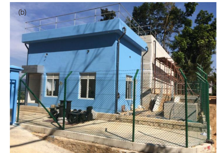
Figure 46: (a) Pihilladeniya Service Reservoir, (b) Uduwawela Service Reservoir
