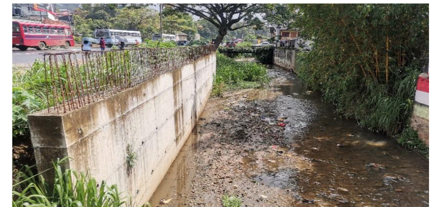
Figure 17: Kandy Meda Ela Rehabilitation Project (in progress)
