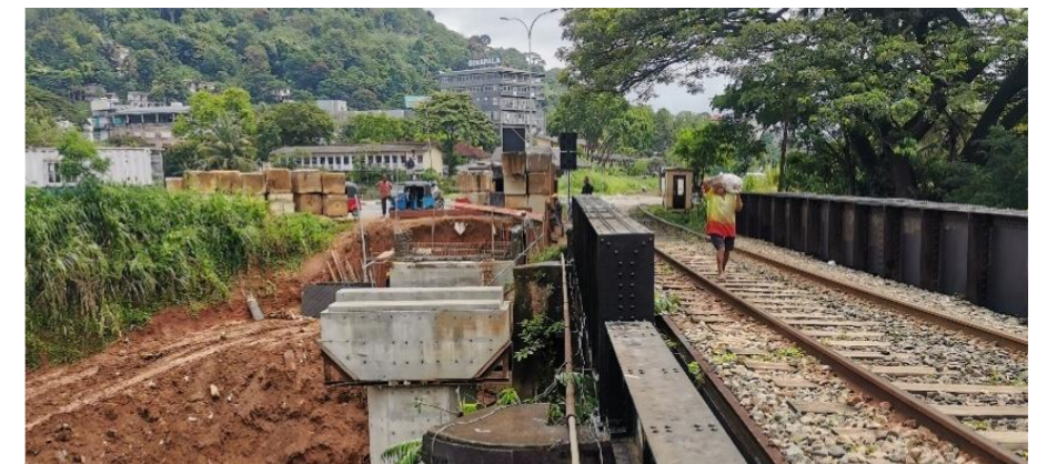
Figure 14: Gatambe Flyover Bridge – works in progress
